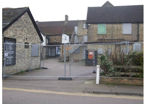
Church Street – fencing across car park entrance
